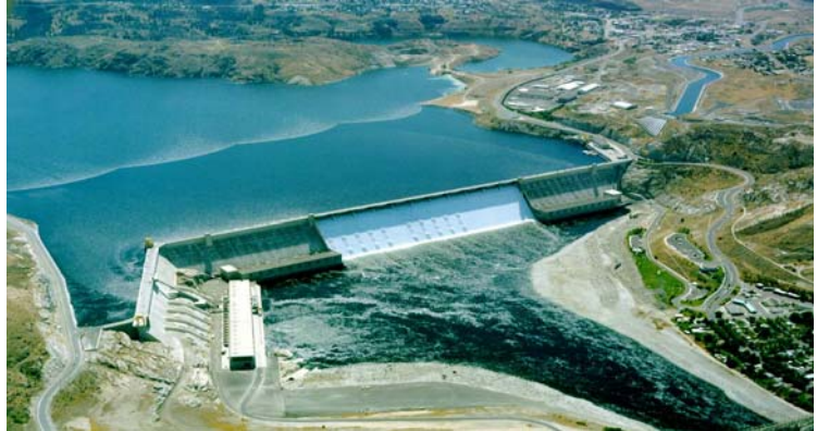
The massive Grand Coulee dam, whose controllable reservoir capability contributes to the uncertainty in regional hydro generation, can generate nearly 6,500 mw of power.
